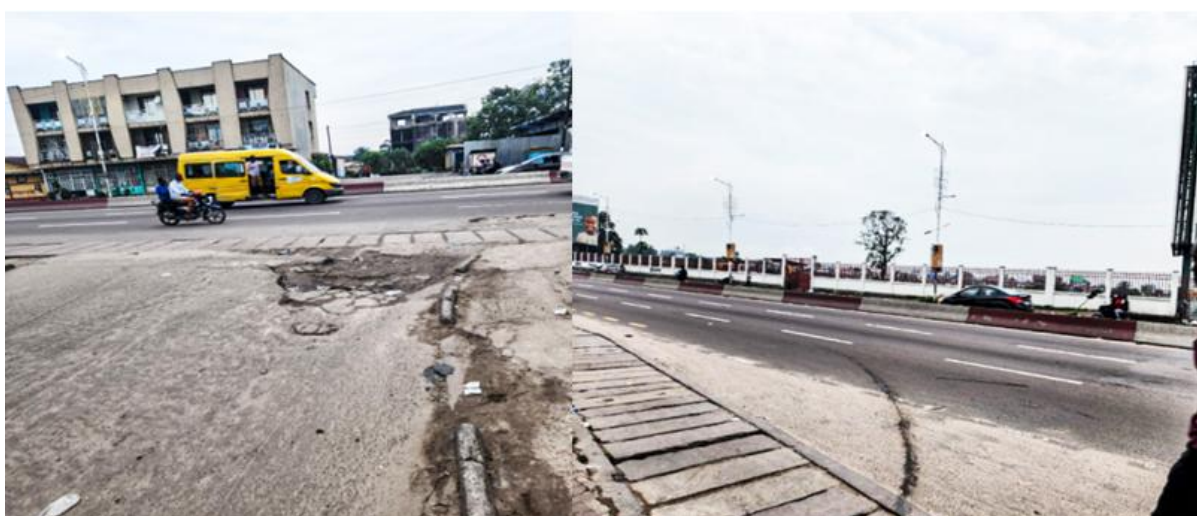
Figure 3: State of some infrastructure completed and handed over in DRC
