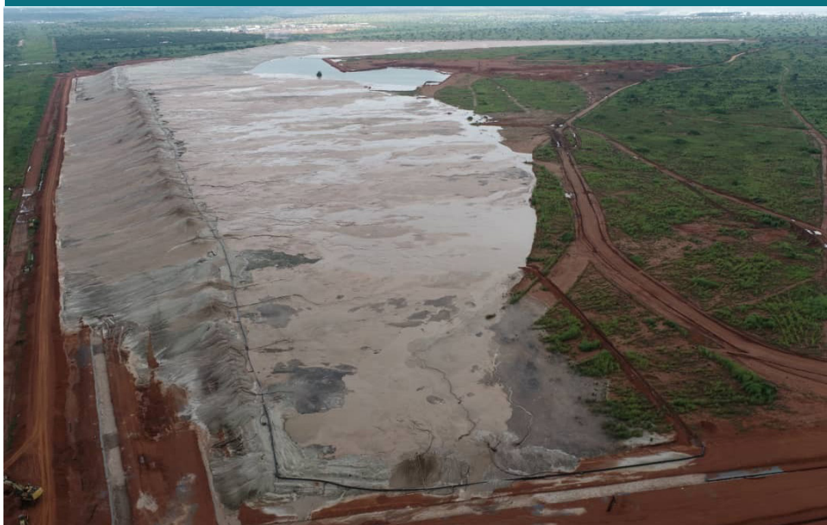
A view of the wastewater spill after the tailings at the Metalkol copper-cobalt mine ruptured
